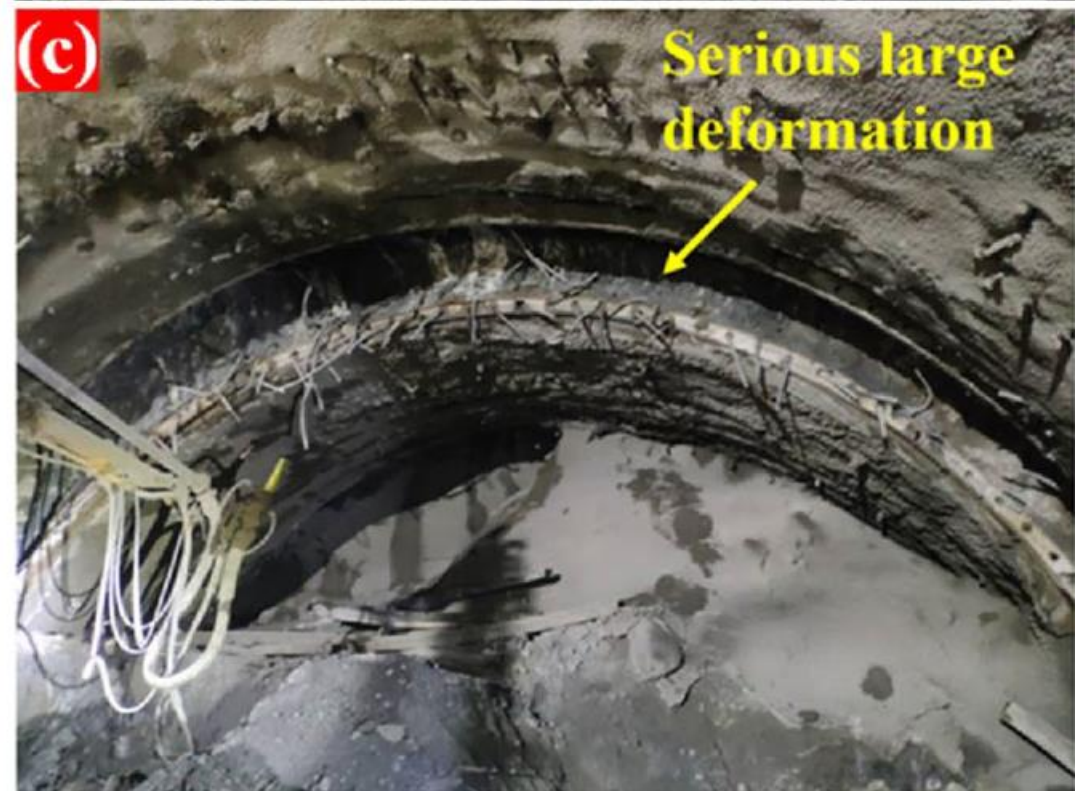
very large anisotropic convergence in Saint-Martin-la-Porte access gallery (after Mathieu 2008)
