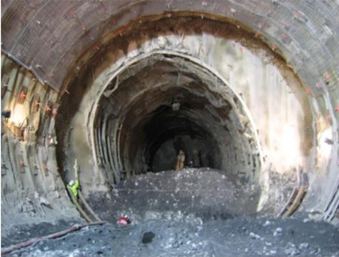
very large anisotropic convergence in Saint-Martin-la-Porte access gallery (after Mathieu 2008)
